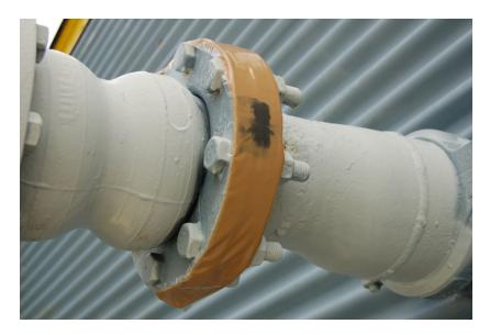
Intellipigment<sup>TM</sup> Hydrogen Leak Detection Tape Discolored Due to Hydrogen Leak
